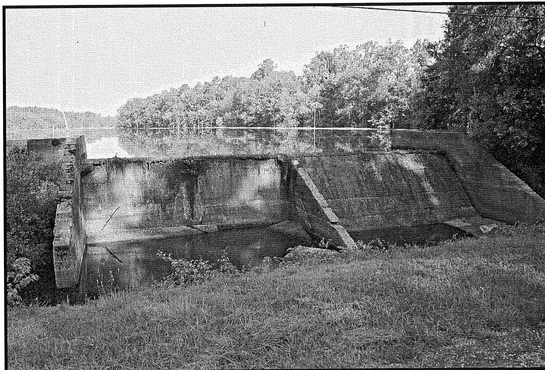
Plate 4: Parker's Mill – looking west toward spillway and pond
