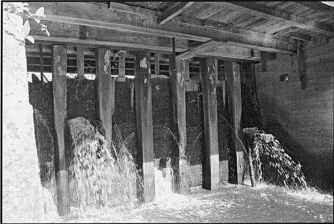
Plate 7: Parker's Mill – spillway under northern block of mill
